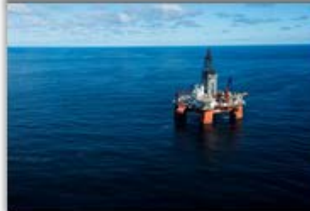
Mobile drilling units
