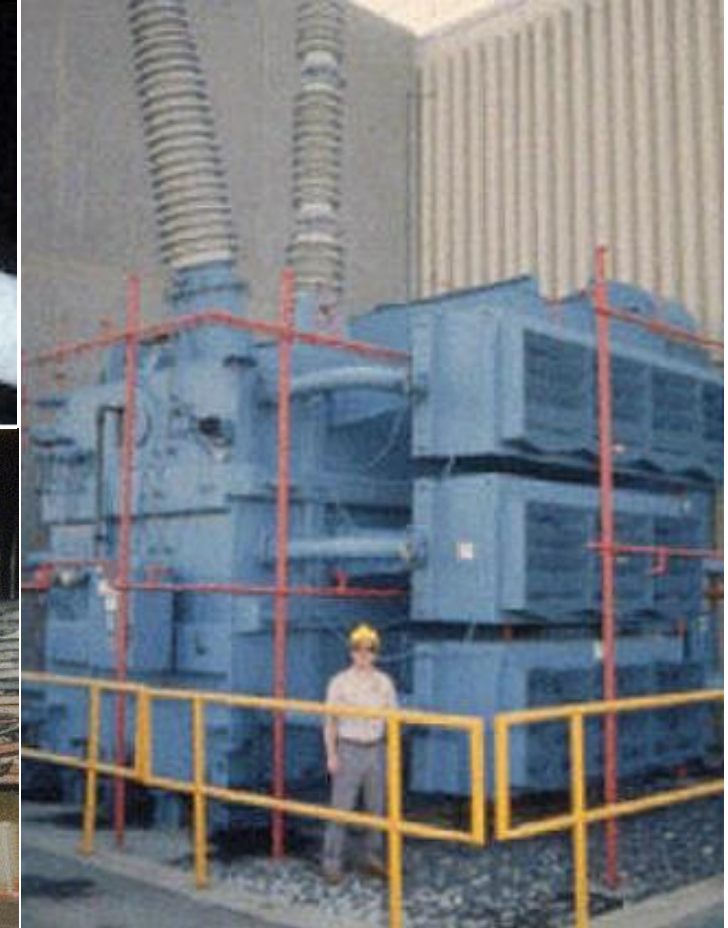
Salem Nuclear Plant GSU Transformer damaged by the GMD event of March 1989. (Photos courtesy of PSE&G.)
