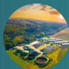
Waste to Energy
